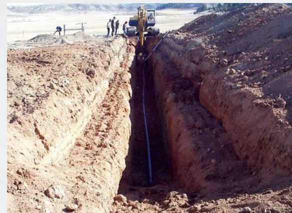
(U) Excavator Digging Large Trench For Utility Installation
