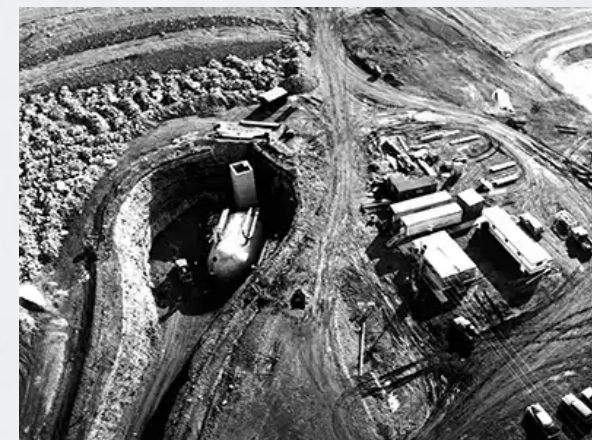
(U) Construction at MMIII Launch Facility
