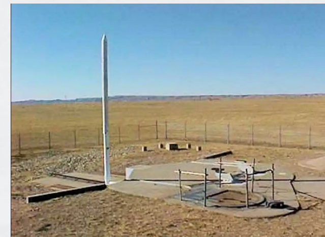
(U) Minuteman III Launch Facility
